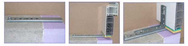
The U-Bar is fixed to the concrete floor using a Heavy-Duty Dowel .
