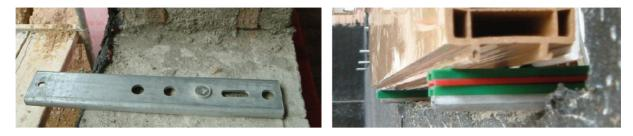
In case of construction zones with insulation, a connecting angle is used for the connection between the window and the U Bar anchor. The angle is fixed to the U Bar anchor with two Drilling Screws.
