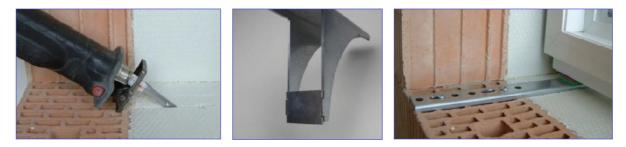
Cut clear the mounting position at insulation area.
