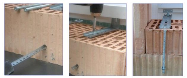
Drill a Ø10 mm hole at least 80 mm beneath the anchor. Then insert the Brick Perforated Rail using the hammer.
