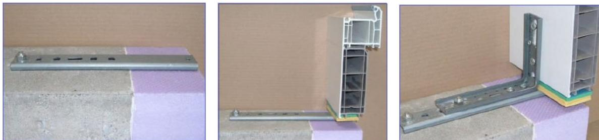
The U-Bar is fixed to the concrete floor using a Heavy-Duty Dowel .
