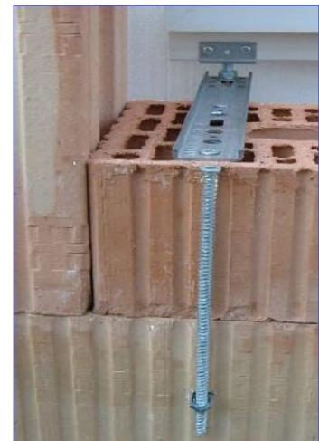
Drill a Ø10 mm hole at least 80 mm beneath the anchor. Then insert the Brick Perforated Rail using the hammer.
