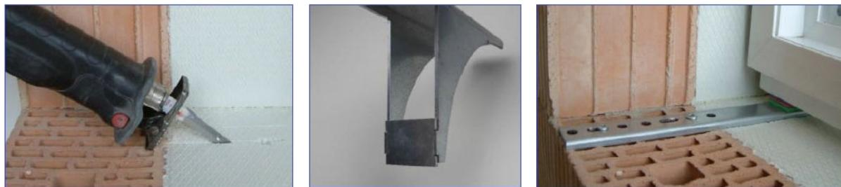
Cut clear the mounting position at insulation area.
